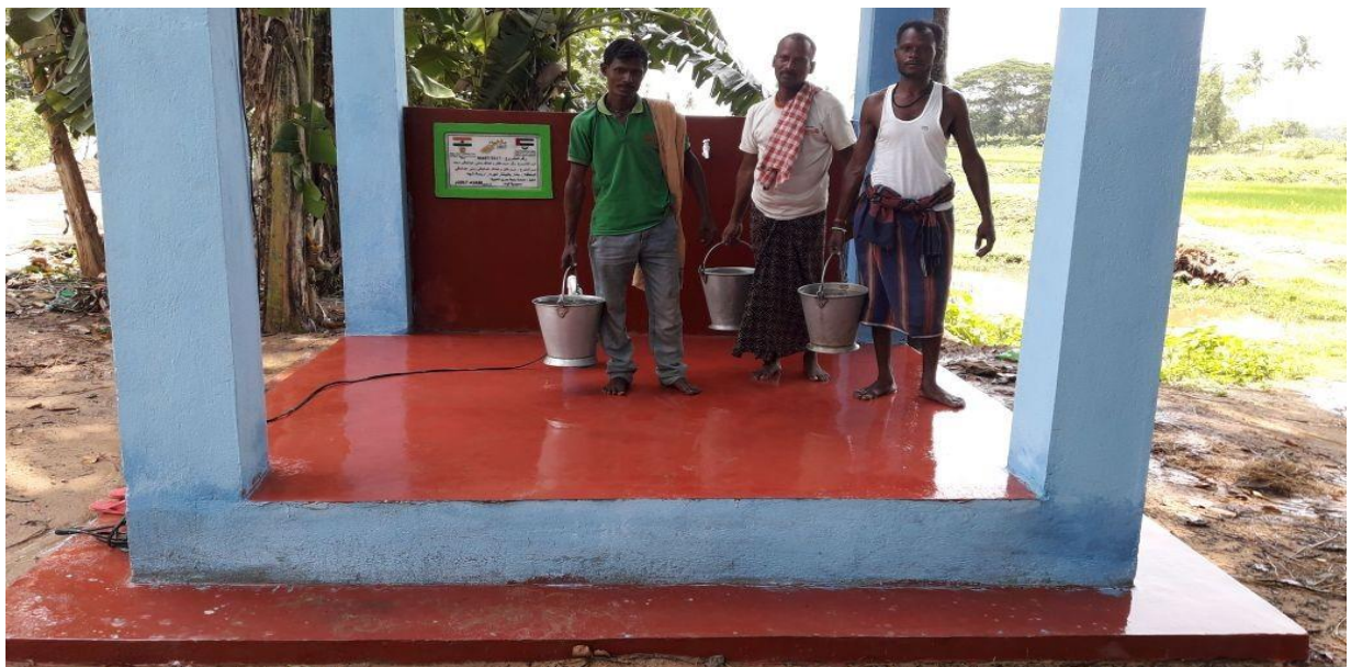
ELEVATED WATER STORAGE TANK
